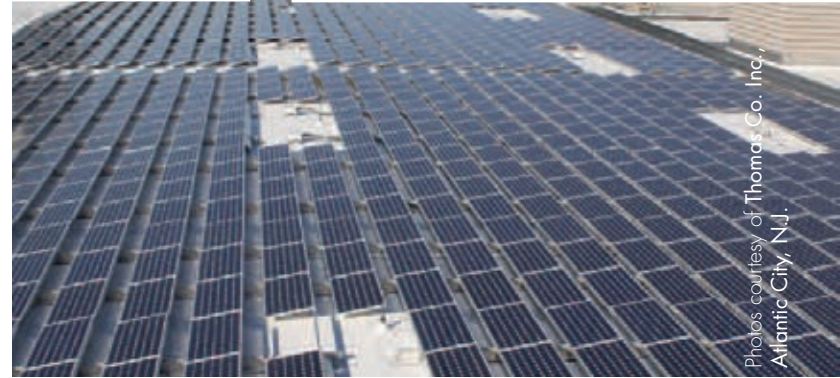
Clockwise from top left: the Atlantic City Convention Center's existing built-up roof system; Thomas Co. installed a GAF Materials white EverGuard TPO membrane; crew members install SECUROCK Roof Board with OlyBond500 adhesive; rack-mounted monocrystalline PV panels on the convention center's roof; the facility's new white TPO roof system before solar array installation
